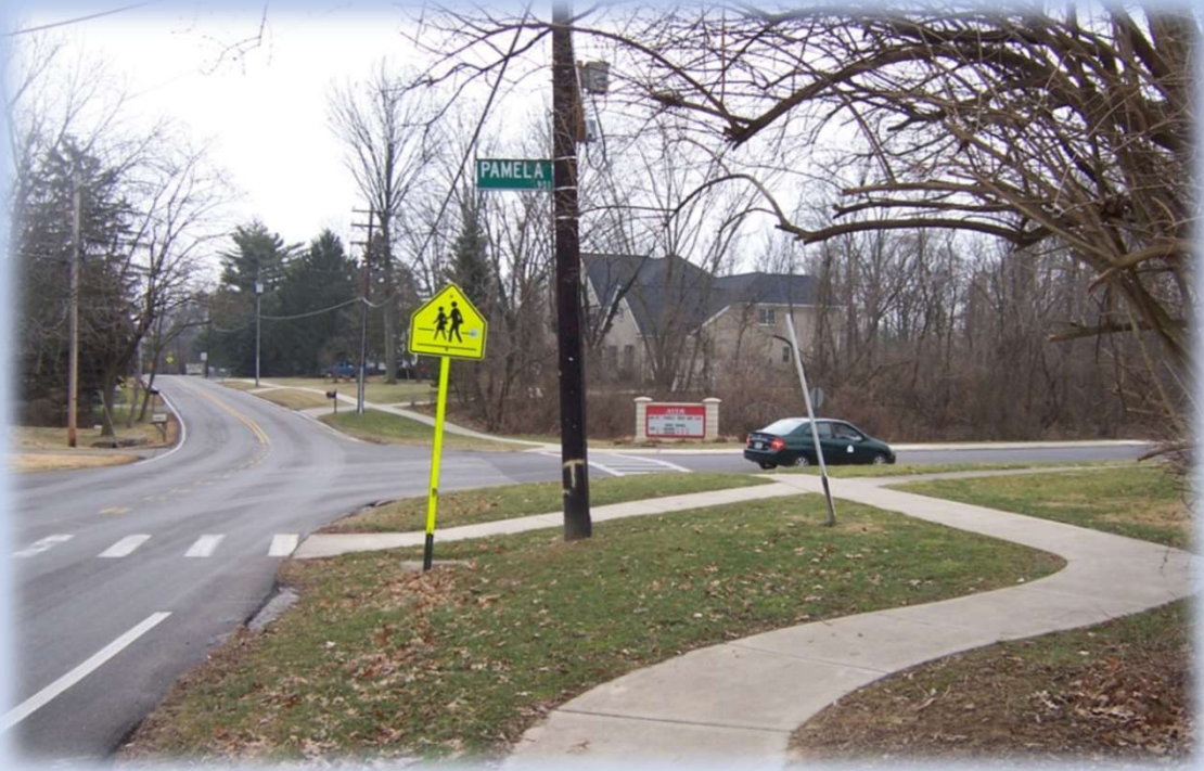
Improved visibility of crosswalks at the Forest Road intersections of Pamela Road and Nottingham Drive (where decorative treatment was tested)
