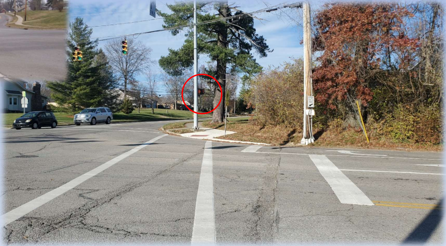
Pedestrian countdown signals at Nagel Road and State Avenue and relocation of crosswalk/ramp across Nagel driveway for sight distance and pedestrian safety
