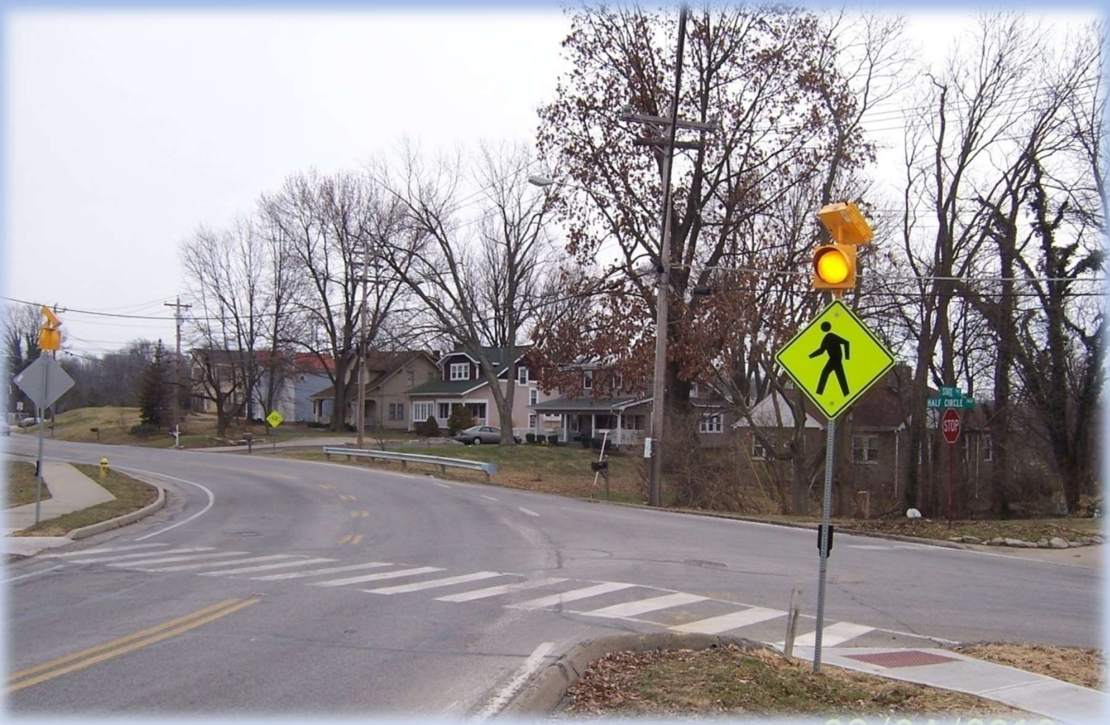
Pedestrian-activated crossing warning lights at crosswalk of State Road and Half Circle Drive (library)
