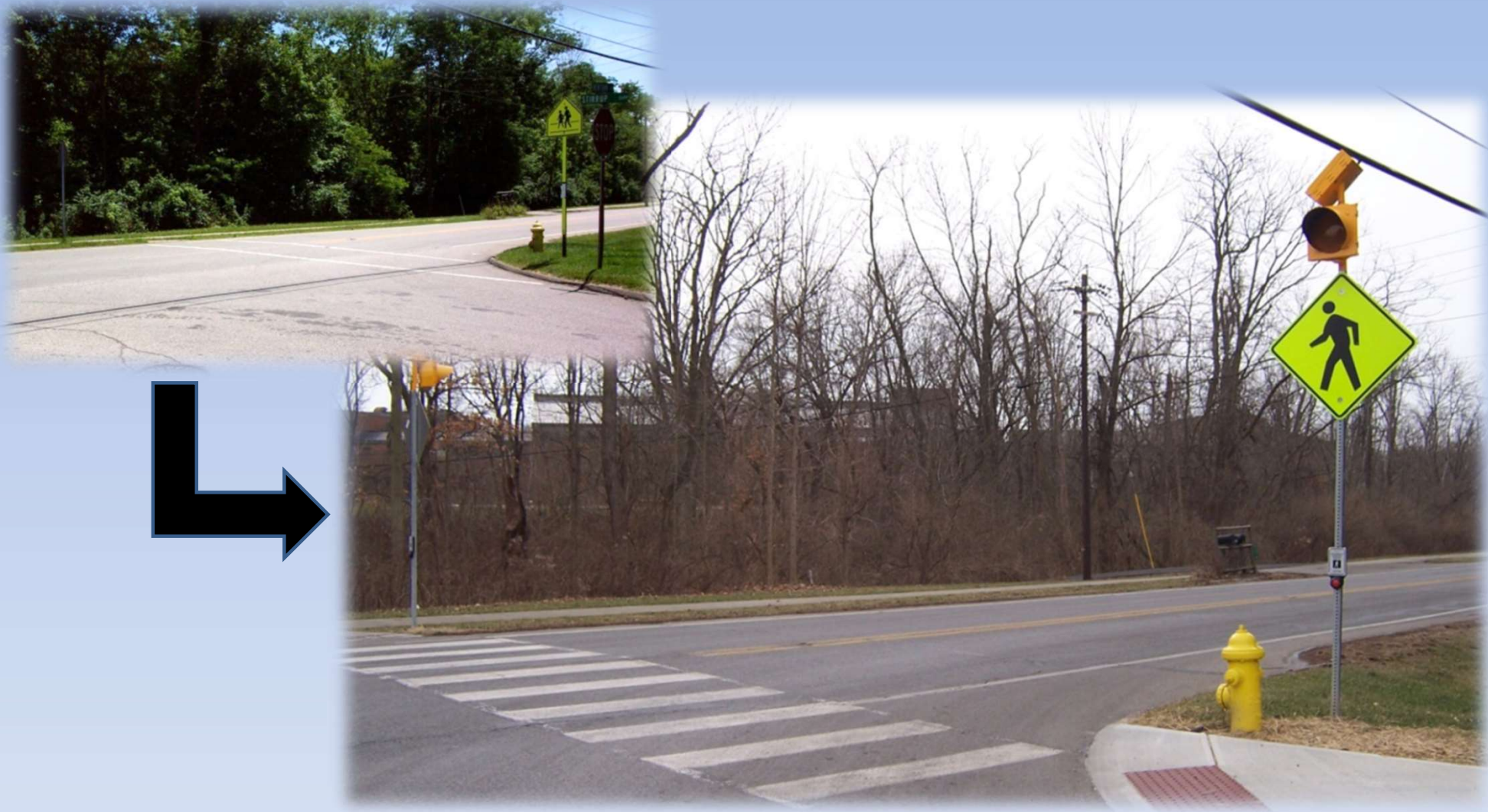
Pedestrian-activated crossing warning lights at crosswalk at Newtown Road and Stirrup Drive and sidewalks on Newtown Road to schools and Five Mile Trail area
