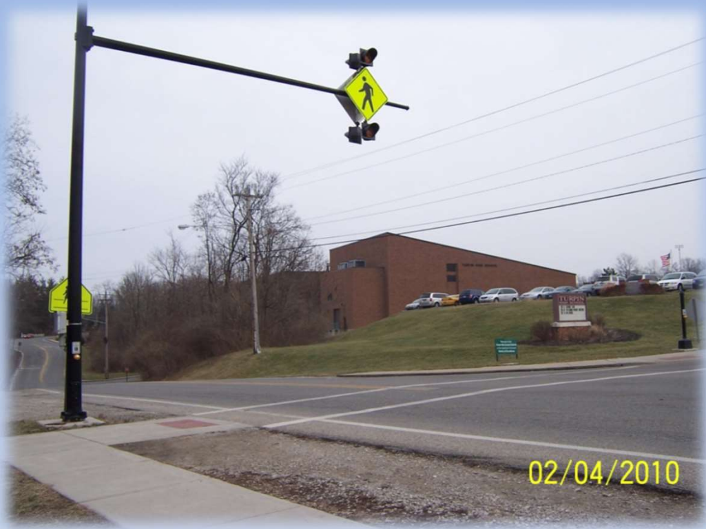
Relocated crosswalk to school entrance with pedestrian activated crosswalk flashing sign and lighting
