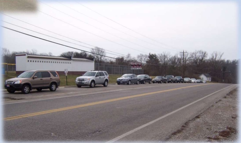
Modified parking on Bartels Road (perpendicular to parallel) and widened roadway to accommodate PM traffic staging on northbound Bartels
