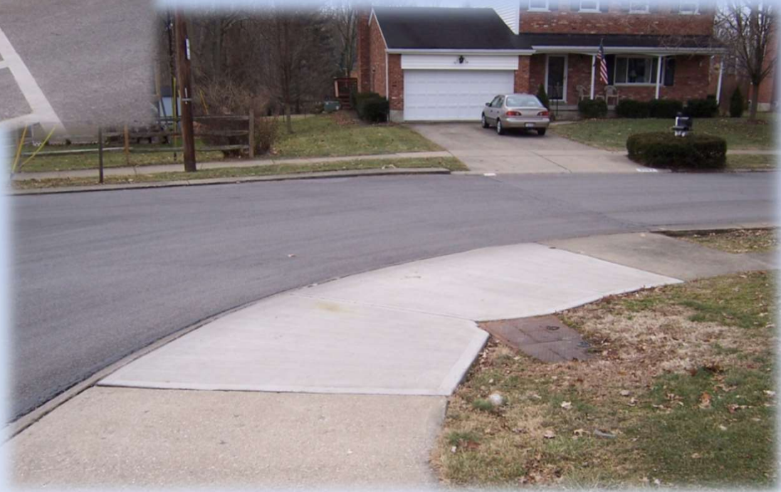
Replaced deteriorated sidewalk blocks and handicapped ramps around the school
