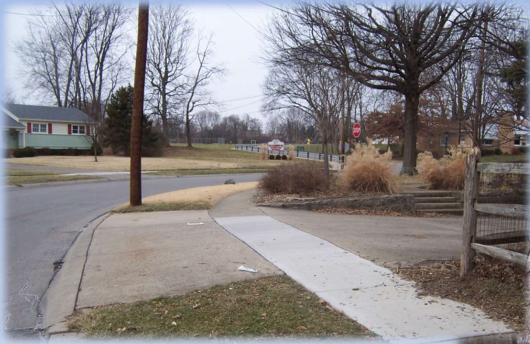
Replaced deteriorated sidewalk blocks around the school
